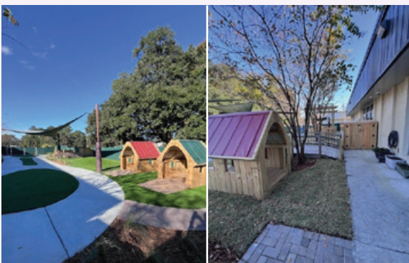
Above pictures showcase the updates and improvements completed to fix drainage complexities and create a safe playground for teammate childcare meeting ABC Quality rating requirements
